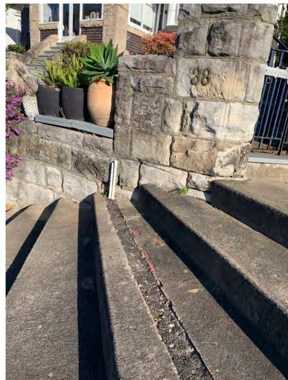
Figure 30. Dudley Street Name embedded in concrete has been cut through for installation of services
